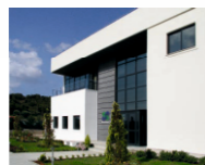
ATTICA Area Panormos, 19500 Lavrio Attiki - Greece
