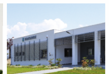
NORTHERN GREECE Lakkoma Industrial Area Halkidiki, 630 80
