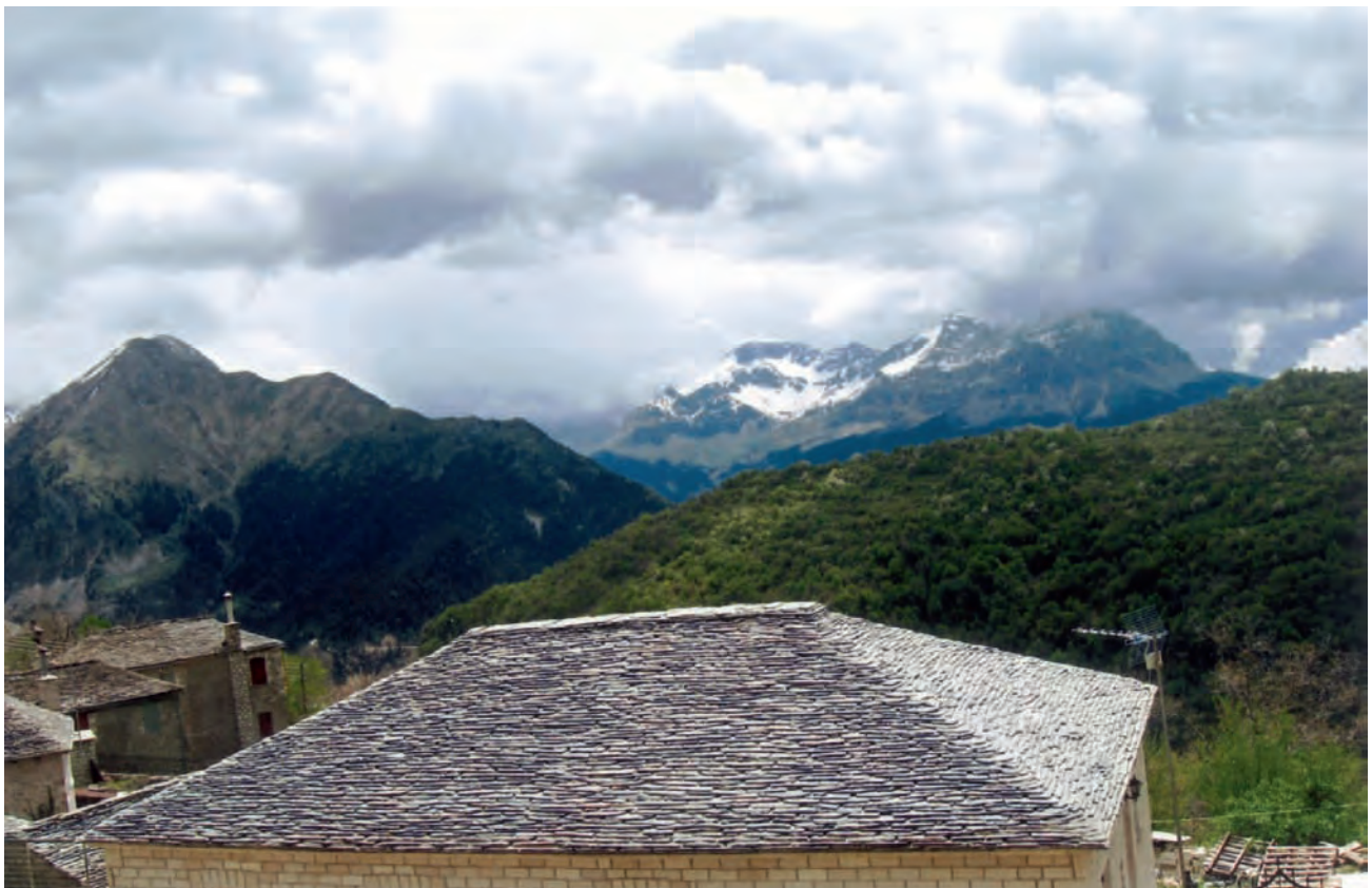
A traditional highland village, Kalarrytes, near Ioannina NW of Greece, where Mr C. Voulgaris the great grand father of the owners of the well-known synonymous jewelry stores was born. Notice the handsome stone-slate-domed roof. One of the crowns of mt. Tzoumerka 2.112m is seen at the background. Sent by Mrs. A Papatriantafidou MA, Thessaloniki.
