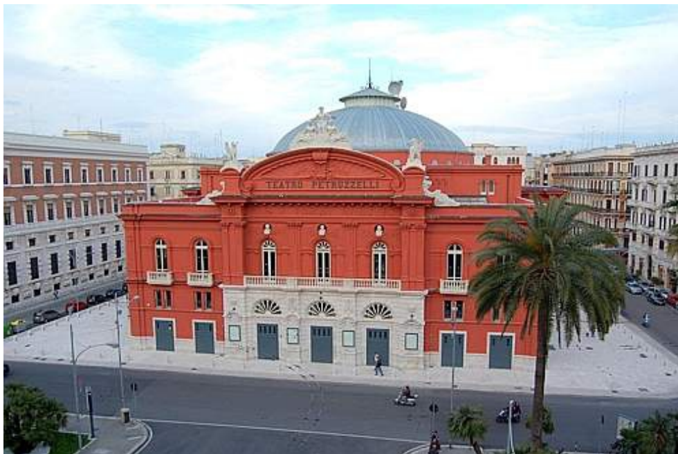
The Petruzzelli Theatre, named after the Petruzzelli brothers, who provided the funding for it, Province of Bari, Italy.
